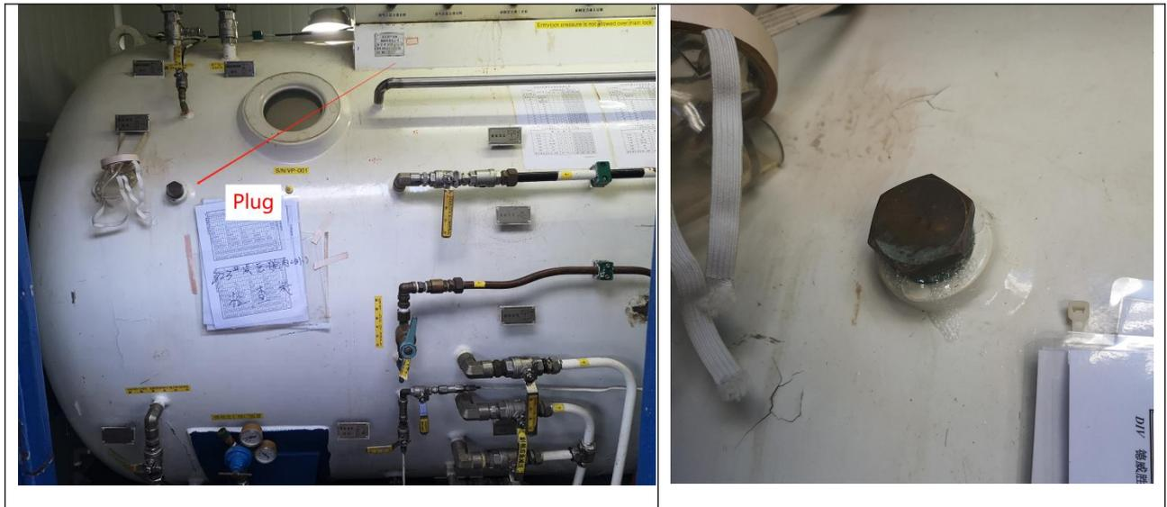
Fig. 10: Plug and when it leaked slightly
