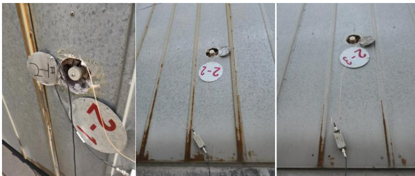
Site sensor partial installation diagram
